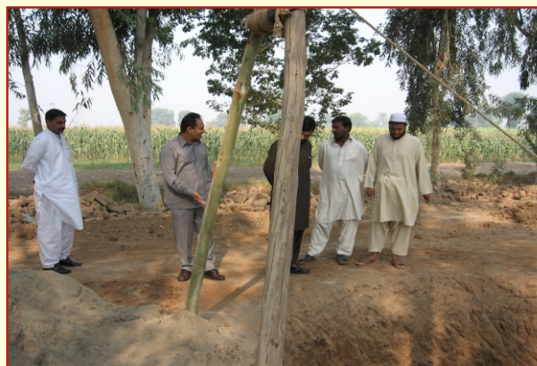
Digging of well
